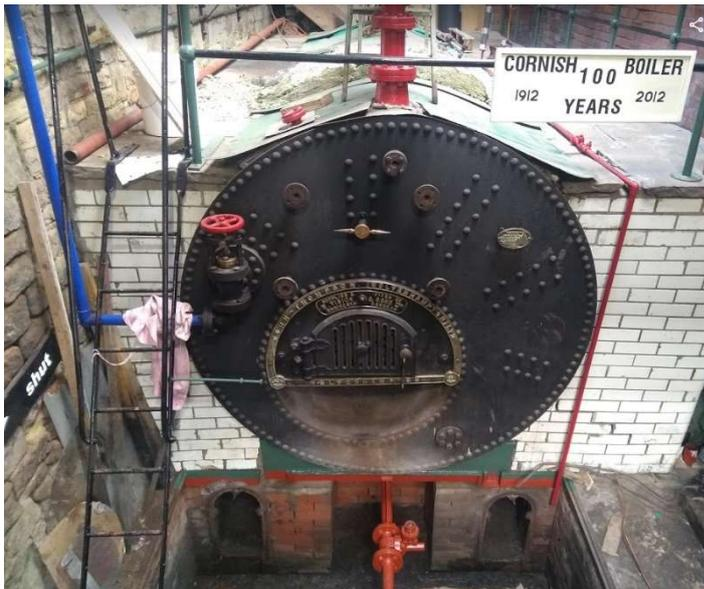
If you look at our Cornish boiler, shown here stripped down for its winter inspection, you will notice that the fire-tube is slightly offset from the centre. Although unusual, it is made that way to facilitate cleaning the bottom of the shell on the water side, and for the better circulation of the water as it becomes hot.
