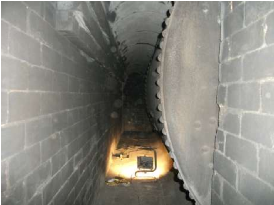
1 Inside of the side flue of the Cornish boiler
